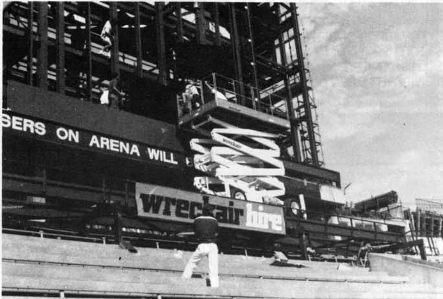
Modules being lifted into place using Wreckair scissor and platform combination.
